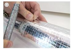
The pipe shell must additionally be secured with soft-galvanized binding wire. duotec: minimum 6 windings per metre; stone wool: 5 windings per metre.
