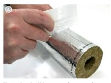
The bonding should be as crease-free as possible. The bonded overlap strip must be pressed on smoothly and firmly with an insulating spatula.
