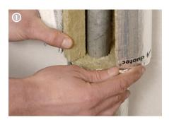
The **pipe shell** with aluminium facing is slit on one side and can be opened up to wrap around the pipe to be insulated.
