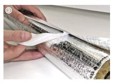
Remove the protective film from the factory-applied self-adhesive overlap and seal the longitudinal slit.
