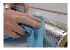
Before closing, the . pipe shell must be pressed together to ensure a precise fit. Ensure that all adhesive areas are free of dust, grease and dry before applying the adhesive tape!
