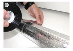
Cross joints of the shells must be laid without joints and additionally secured with suitable adhesive tape from the manufacturer. Adhesive tapes should generally be pressed on smoothly and firmly with an insulating spatula.
